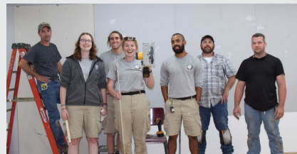
Renovations at Swink Early Learning Center site NCCC team and LDCAA WX staff
